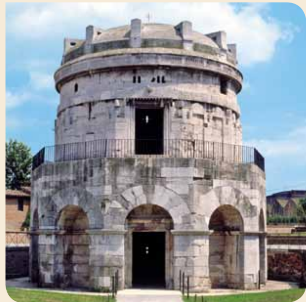
Mausoleum of Theodoric in Ravenna, Italy. Built by the Ostrogoths around the year 520.
